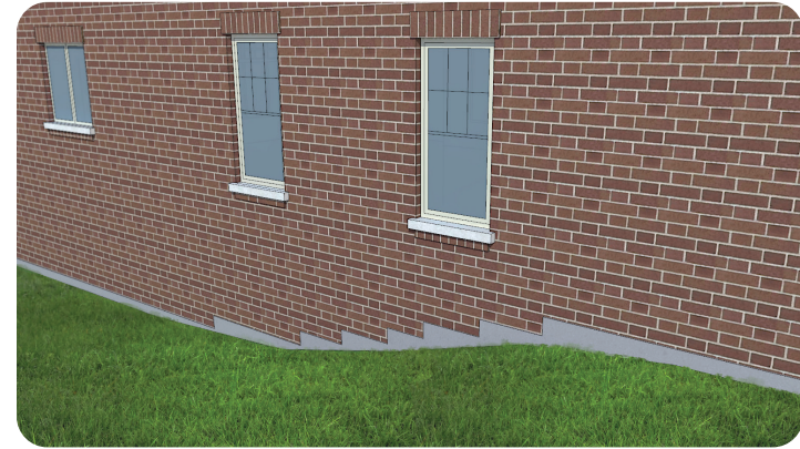
Foundation Wall at Sloping Grade
