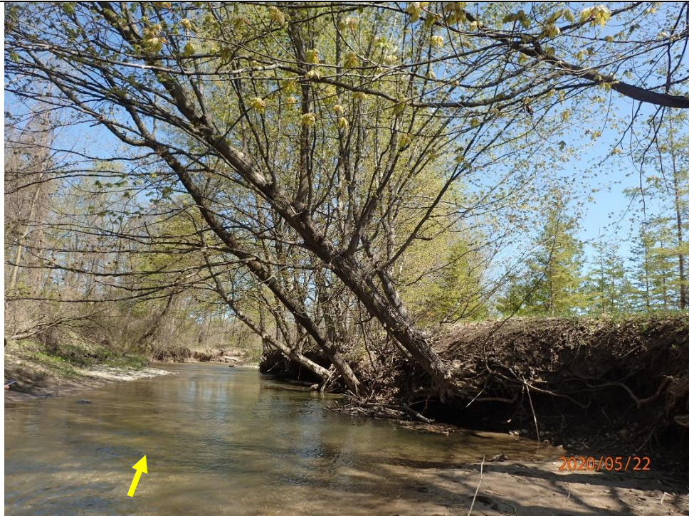
Photograph taken further downstream, leaning and fallen trees were commonly identified along the reach, indicating evidence of channel widening.
