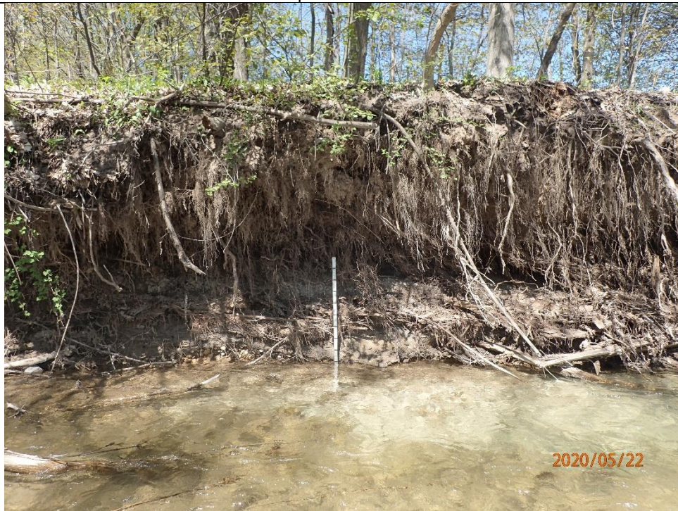
Photograph taken looking at the left bank. Large undercuts were common (approximately 1.65 m in depth), this is an indication of erosion leading to channel widening.
