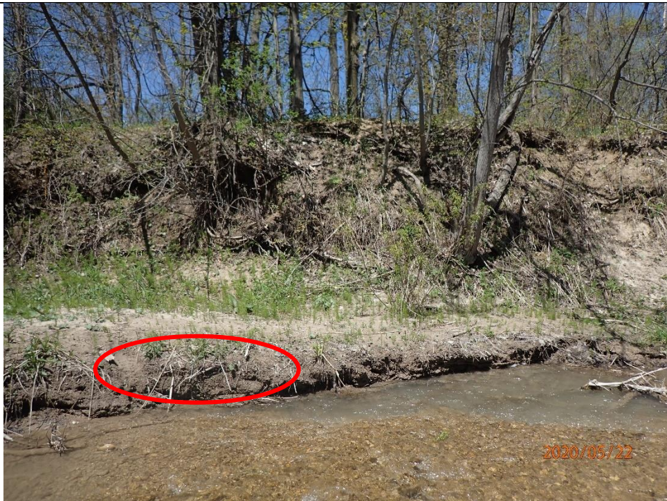
This photograph illustrates a well-vegetated, confined section of the watercourse. Erosion scarring on the base of the channel bank is indicative of widening processes.
