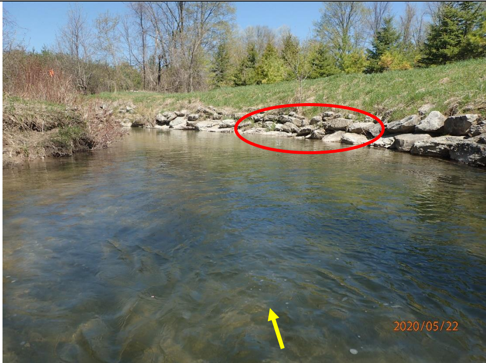
Photograph looking downstream, bank stabilization (cobble and boulders) were present along the outside of meander bends to prevent erosion.
